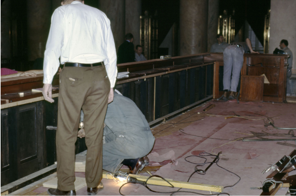
Photograph of the bench in the Supreme Court Courtroom in January/February 1972, when it was altered to create three angled sections for improved viewing and sound. The authors conclude that the bench change led to fewer interruptions by the Justices, particularly of those sitting at the ends of the bench.
